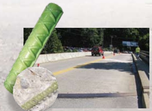
Bridge No. 2953 Coated bars in top and bottom mat.
