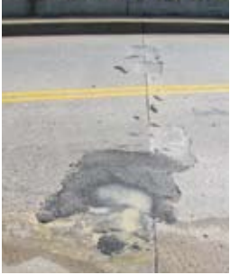
Repair of Span 5 of Bridge No. 2930 containing black bar.
