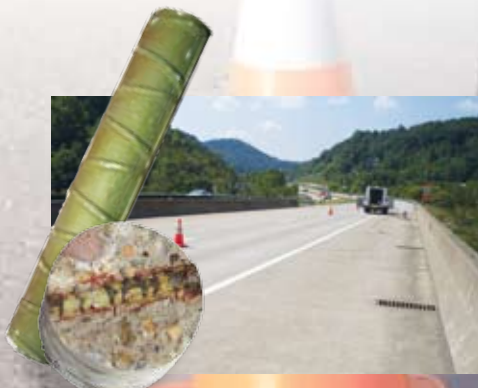
Bridge No. 2672 S Coated bars in top mat only.
