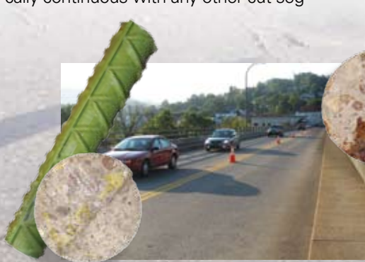
Bridge No. 2930, Spans 1-4 Coated bars in top and bottom mat.
