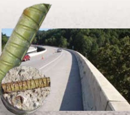
Bridge No. 2668 N Coated bars in top and bottom mat.
