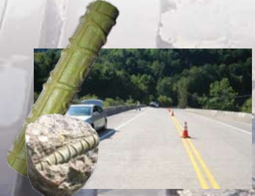
Bridge No. 2673 Coated bars in top mat only.
