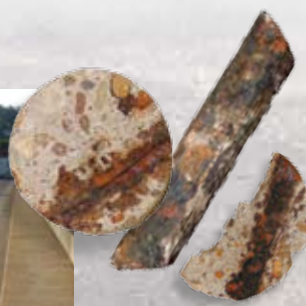
Bridge No. 2930, Spans 5-6 Black bar in top and bottom mat.
