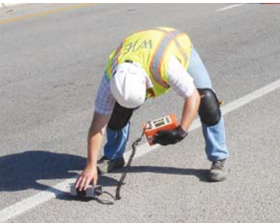
Measuring concrete cover over reinforcing bars.
