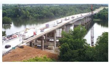
Recently reconstructed I-40 bridge in Oklahoma. Completed in 65 days using 235 tons of epoxy-coated rebar in both decks following a barge collision that collapsed the original bridge.
