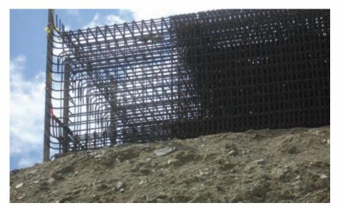
Reinforcing cage for Galena Creek Bridge Arch
