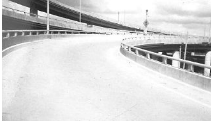
Top Deck of Kentucky Bridge circa 1975
