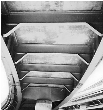
Underdeck of above Kentucky Bridge in 1993
