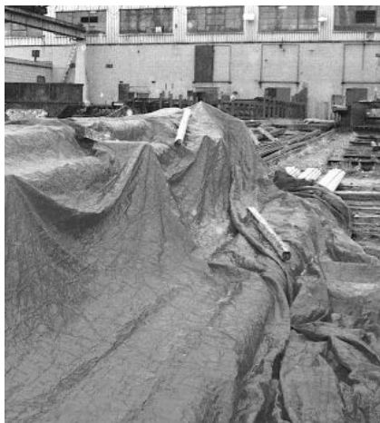
Draped bar bundles in long-term storage
