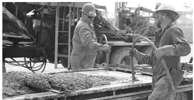
Compaction using non-metallic vibrator heads
