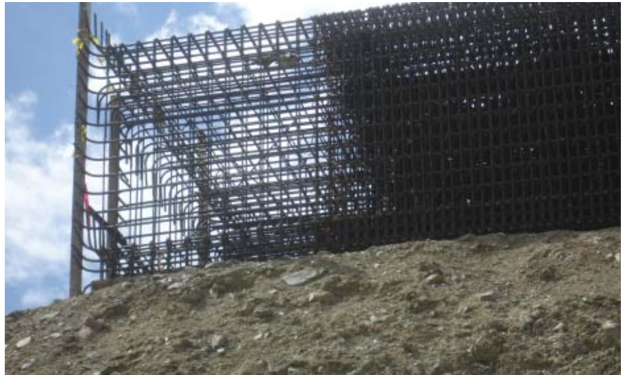
Reinforcing cage for Galena Creek Bridge Arch
