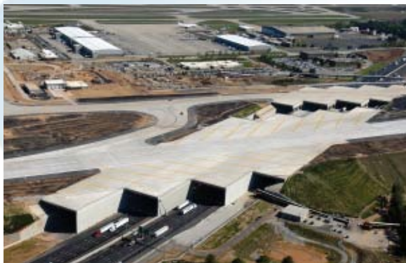
Aerial view of Interstate 285 and box culverts
