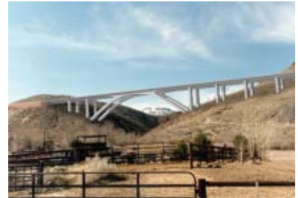
Galena Creek Bridge
