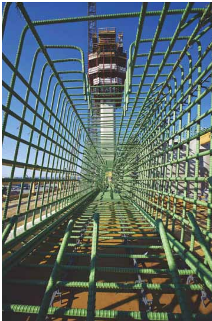
Epoxy-coated reinforcement shown in the Indian River Inlet Bridge. Photo: AECOM.
