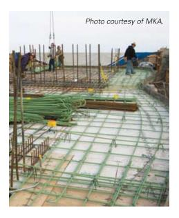
would occur. Approximately 2445 tons of epoxy-coated reinforcing bar was used.
