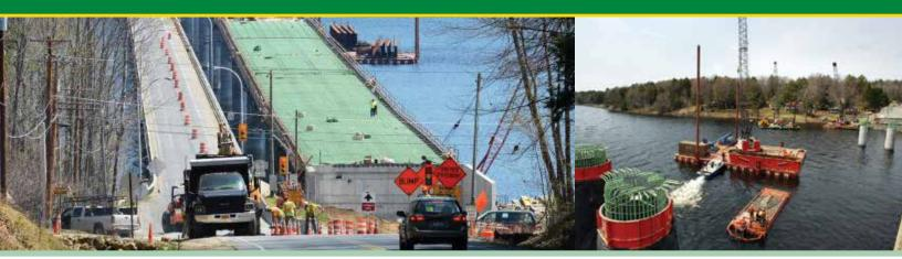
The original Batchellerville Bridge was constructing in 1927 and the deck and railing was replaced in 1982. Due to corrosion the bridge traffic had been reduced to a single lane to limit the amount of load on the bridge. The existing 3000 foot long Batchellerville Bridge carries Saratoga County Route 98 over the Sacandaga Lake and is the only bridge across this lake.
