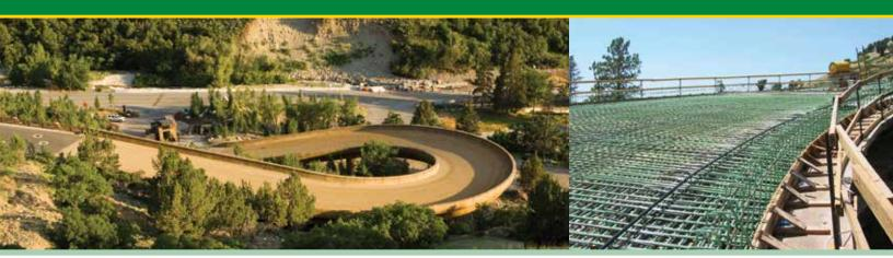
A strong welcoming presence was needed to attract buyers to a new upscale housing community near Utah's Wasatch Mountains, but the difficult terrain created challenges. To meet both functional and aesthetic needs, two reinforced concrete bridges were created, including a five-span, 450-foot-long structure with a switchback curve along an 80-foot radius of the centerline.
