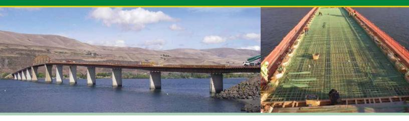
The Biggs Rapids/Sam Hill Bridge (US 97) provides a vital link between Oregon and Washington and in 2009, the bridge was given a more durable concrete deck containing epoxy-coated reinforcing steel (rebar). The previous bridge deck was deteriorating at a rapid rate, requiring excessive and costly maintenance repairs.
