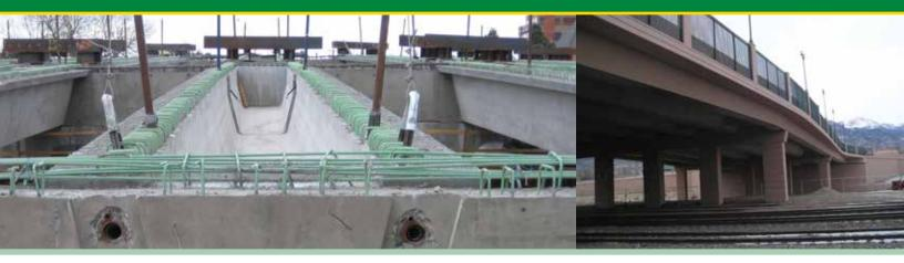
Colorado Springs needed a new bridge to relieve congestion and provide added access to the downtown area as well as project a new welcoming image for the city. These goals were reached with a design that featured a spliced, post-tensioned, precast concrete superstructure with an innovative prestressing layouts and variable cross-sections to accommodate a unique erection methodology. The project was completed in only 10 months.
