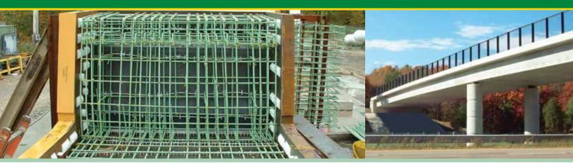
The precast concrete "channel" design for the DCR Access Road Bridge over Route 24 will improve clearance for the heavily traveled road below, complement the surrounding scenic areas and reuse existing materials to reduce waste and lower costs. It also offers significant opportunities for expanding the capabilities of post-tensioned segmental construction.
