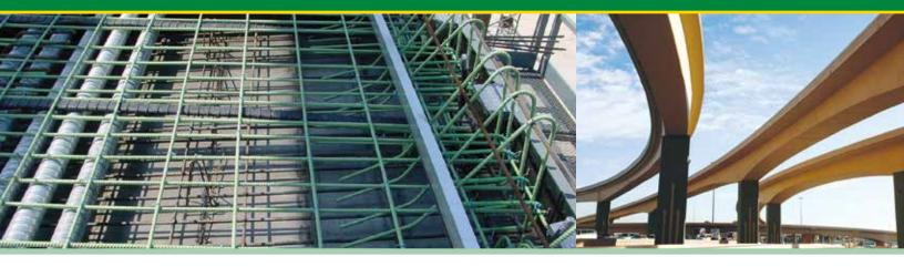
Faster construction and the ability to minimize impacts to traffic were key goals for the construction of concrete segmental ramps on the Dallas High Five project, which consisted of five ramps with span lengths up to 300 ft long.
