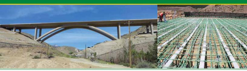
When completed, the twin Galena Creek Bridge on I-580 near Reno NV will be the largest concrete cathedral-arch bridge in the world, measuring over 1,725 feet with a central span of almost 690 feet. This bridge, designed by NDOT, is part of a \$450-million, 8.5-mile-long I-580 Freeway Extension that will help connect Reno and Carson City. Construction on the bridge started in 2003.
