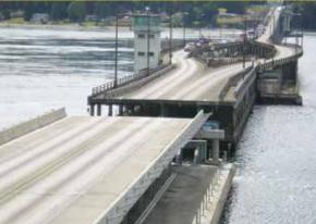
The Hood Canal Bridge carries Washington State Route 104 across Hood Canal connecting the Olympic and Kitsap Peninsulas. The bridge, first opened in 1961, provides a vital link between these two peninsulas, carrying approximately 16,500 vehicles per day. The 7,869 ft long bridge has a 600 ft draw span to allow for shipping.
