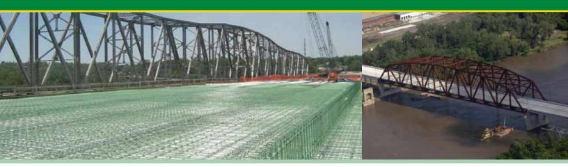
The new 4,300-foot Veterans Memorial Bridge in South Omaha, Neb., replaces a narrow and structurally deficient bridge. The river span is a 625-foot truss to accommodate the 590-foot clear navigation span required by the U.S. Coast Guard. The bridge provides a direct route across the Missouri River to the Omaha Stockyards for livestock delivery trucks.
