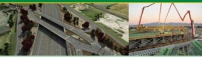
In 2008, a \$172 million project was initiated just south of Salt Lake City, on I-15 as part of a 1-mile reconstruction project. The project is the third diverting diamond interchange (DDI) in the US. These designs reduce the number of accidents that occur and reduce traffic congestion.
