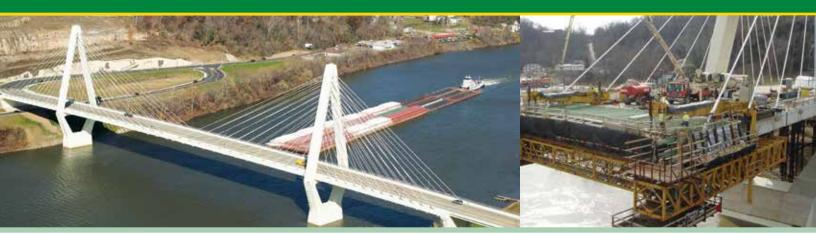
The new Pomeroy-Mason Bridge replaces a structurally deficient steel-truss design to carry Ohio SR 33 over the Ohio River. The cast-in-place, segmental, cable-stayed bridge represents a unique partnership, as it was built by the Ohio Department of Transportation and then turned over to West Virginia Department of Highways to maintain.
