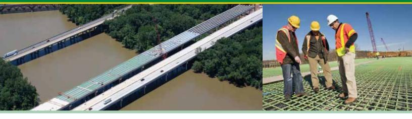
In 2013, NCDOT opened the new I-85 Yadkin River Veterans Memorial Bridges, which replaces the original bridge built in 1955. The new bridge, consisting of eight bents and nine spans, was built using top-down construction that eliminated the need for a temporary work bridge and reduces the impact to the environment. Epoxy-coated reinforcing steel (ECR rebar) was used in the deck construction of the structure to provide corrosion protection to the reinforcing steel.
