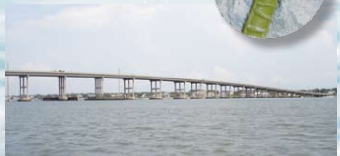
Atlantic Beach Bridge Atlantic Beach, North Carolina
