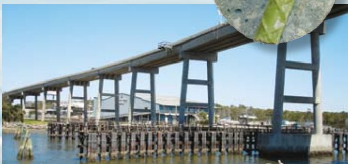
Holden Beach Bridge Holden Beach, North Carolina
