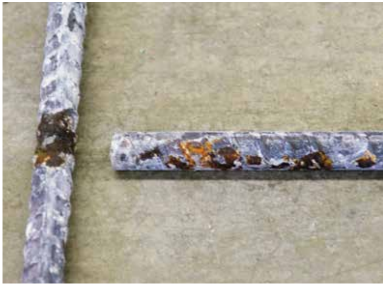
Close-up of corrosion on LLC A1035 bar (cracked specimen).
