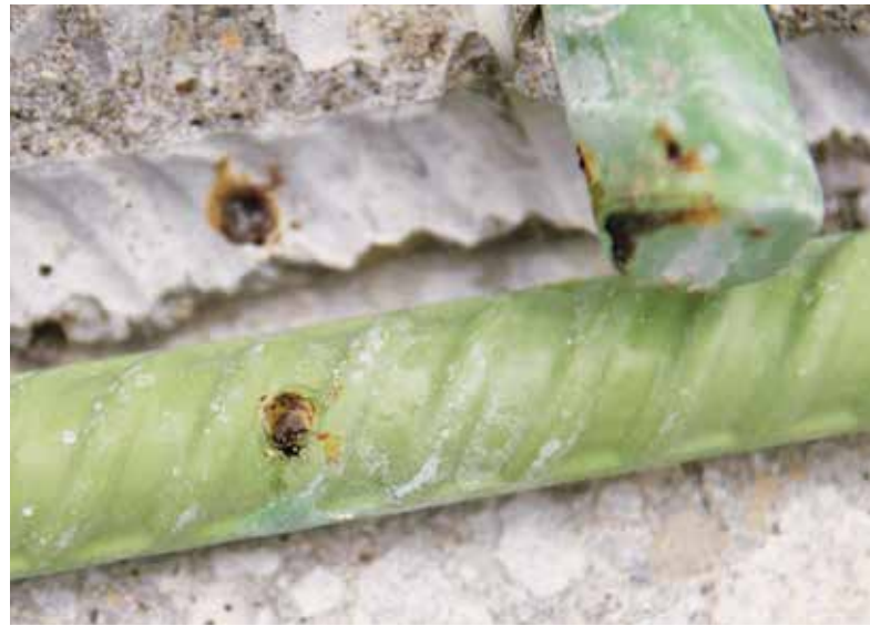
Close-up of corrosion on epoxy-coated A775 bar (cracked specimen).
