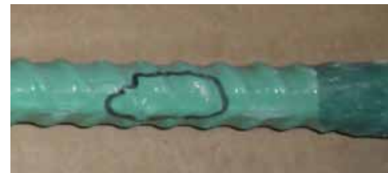
Figure 5 Epoxy-coated reinforcing steel (pinhole) in OPC after impressed current test.
