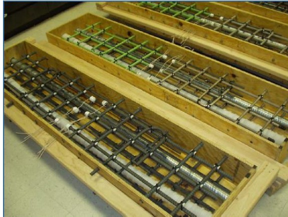
Fig. 6: Concrete slabs prior to casting of concrete (Lee 8 )
