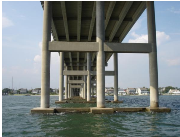
Figure 1: Bridge at Atlantic Beach, N.C.
