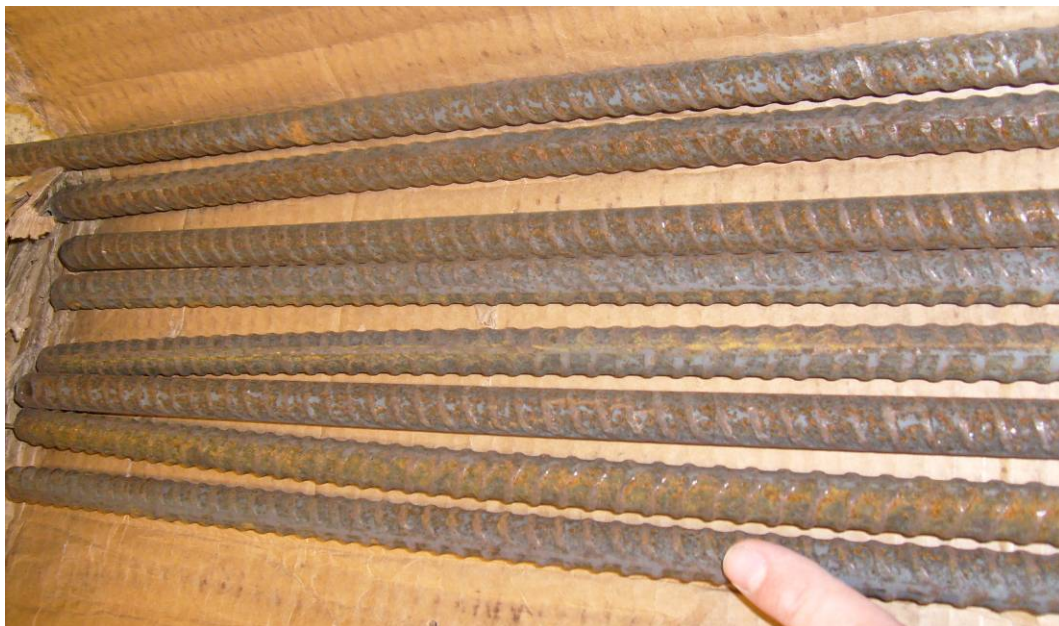
Figure 1: A1035 steel in the as-received condition exhibit corrosion on the surface of the bars.
