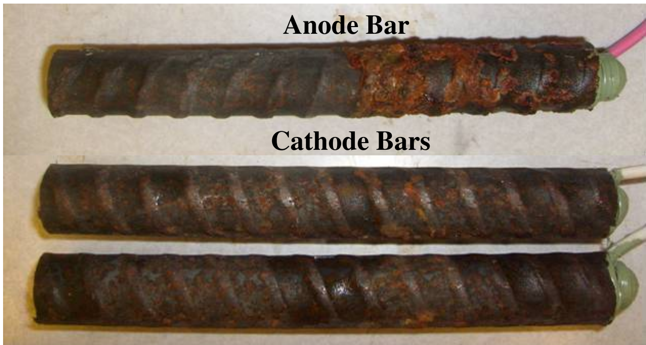
Figure 21: A1035 steel. Specimen 3, side B one week after removal from solution, after rinsing. Specimen exhibits significant corrosion above the liquid level.
