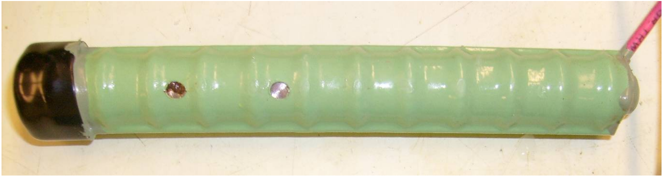
Figure 38: Corrosion typical of that seen on 0.83% damaged area ECR at conclusion of the test. Specimen 5, side A.
