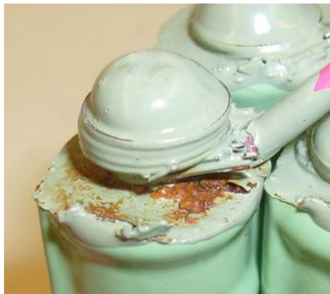
Figure A7: Undamaged ECR, specimen 4 anode exhibits significant steel corrosion at the electrical connection.
