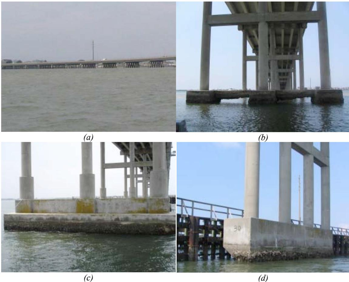
*Figure 32. Atlantic Beach Bridge substructure configuration: a) prestressed piles (Bent 1-14 and 44-48); b) pile caps with thin strut (Bents 15-25 and 34-43); c) pile caps with shafts (Bents 26-28 and 31-33); d) pile cap with a haunch (Channel Bents 29 and 30).*
