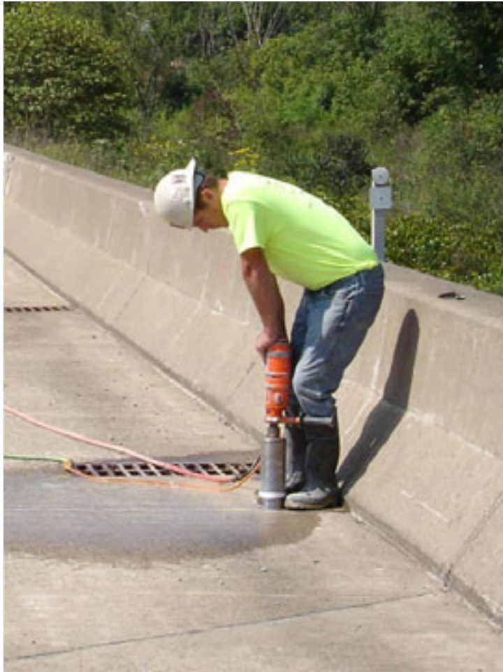
Figure 2. Core sample extraction.
