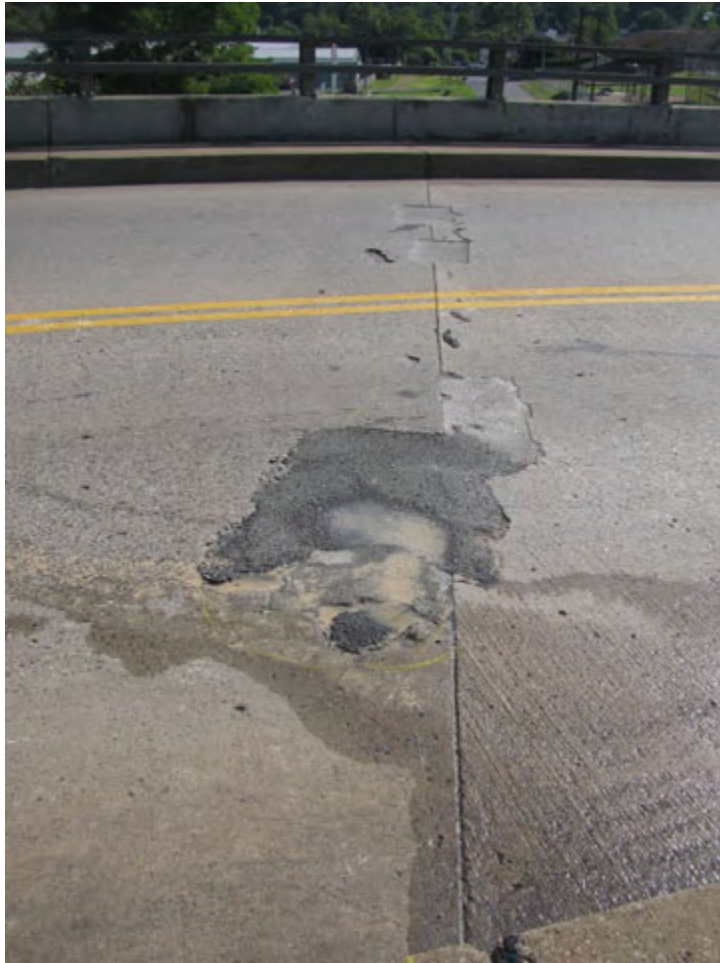
Figure 23. Repair on Span 5 of Bridge No. 2930.
