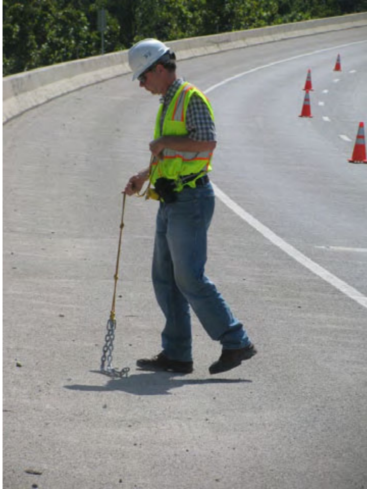
Figure 1. Mechanical sounding to identify delaminations.
