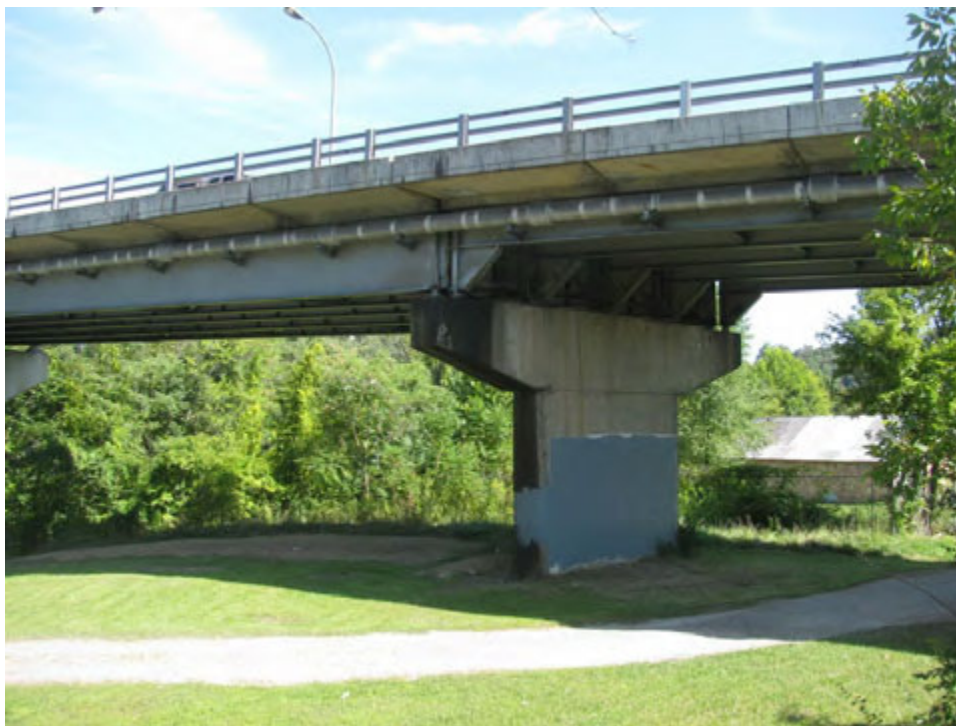
Figure 21. West side of Pier 4 of Bridge No. 2930.
