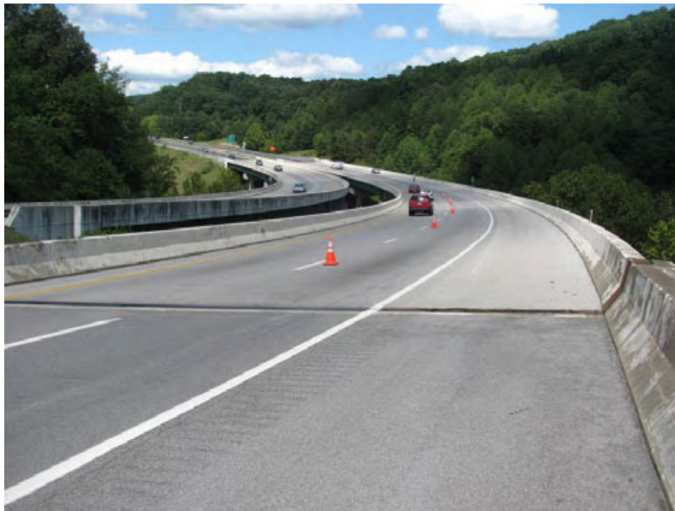
Figure 8. Bridge No. 2668N
