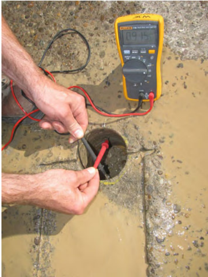
Figure 3. Measuring continuity (electrical resistance) of reinforcing bar mat.
