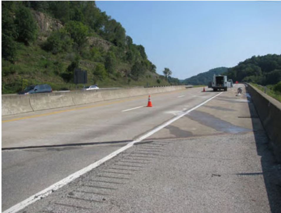
Figure 11. Bridge No. 2672N.
