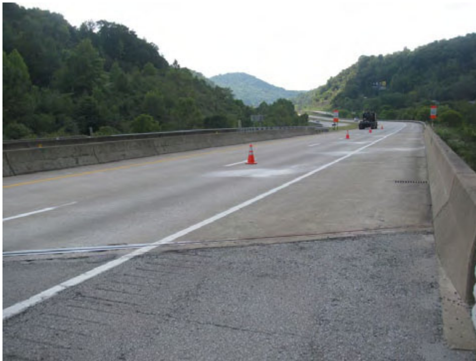
Figure 12. Bridge No. 2672S.
