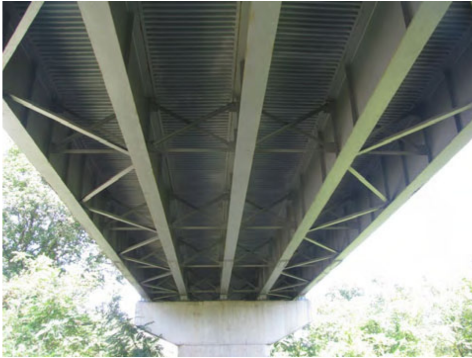
Figure 22. Stay-in-place forms in Spans 1-4 of Bridge No. 2930.
