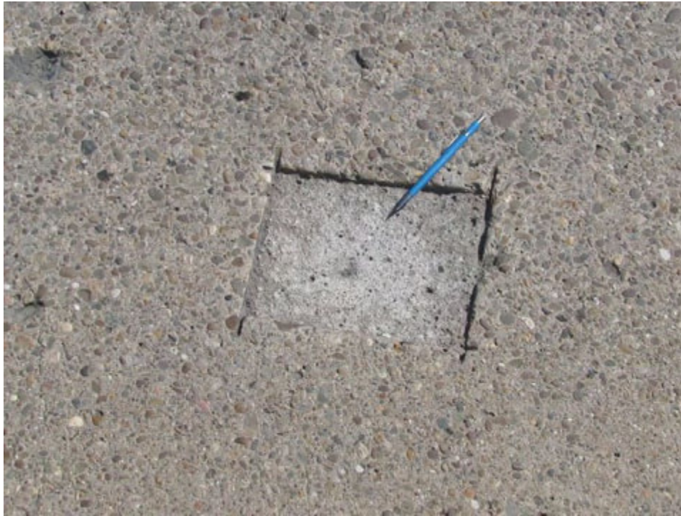
Figure 24. Isolated repairs on Bridge No. 2930.
