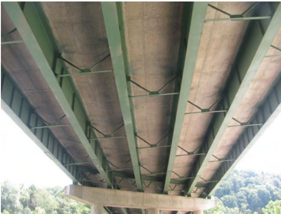
Figure 19. Underside of Bridge No. 2673.
