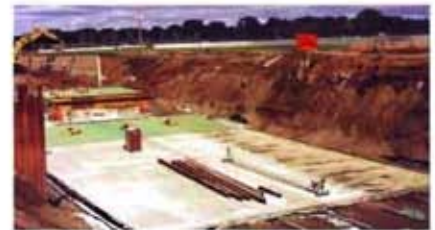
Bottom slab construction
