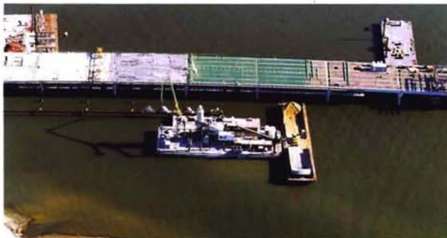
Construction of west side approach spans
