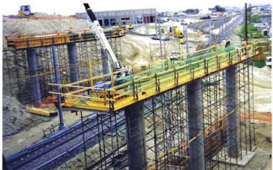
Pier cap construction
