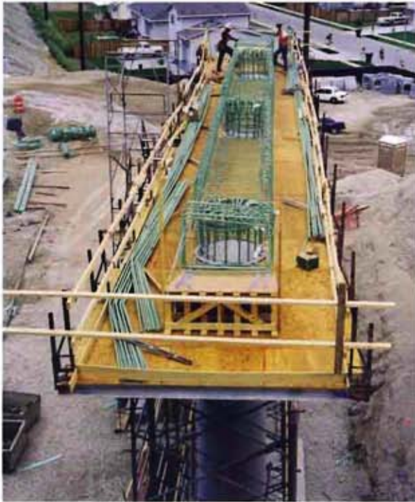
Bridge pier cap reinforcing steel
