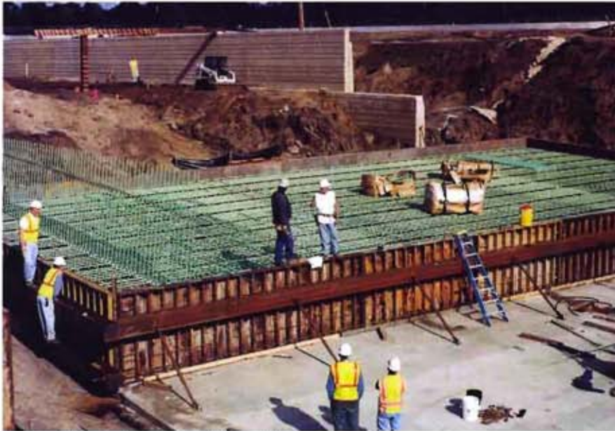
Construction of airport tunnel's base slab
