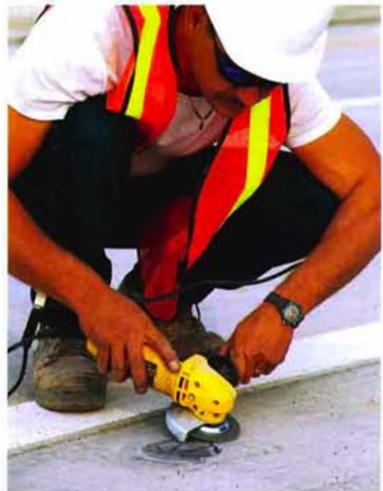
Installation of anti-icing system in bridge deck
