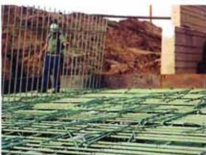
Placement of reinforcing steel for tunnel base and wall
