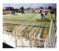
highway in the decades ahead was made possible because the vital components of the concrete structures were protected against corrosion with epoxy-coated reinforcement.
