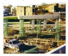
To achieve the extended service life required by the designers, 2,500 tons of epoxy-coated reinforcing bars were used. This major highway rebuilding project along a 4.7-mile stretch of M-39 from I-94 to M-153 includes improvements to fifteen ramps, six bridges plus new lighting and signage. The six
