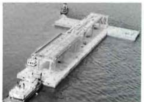
Football field size pontoon with superstructure/roadbed is floated up Puget Sound to bridge site.
