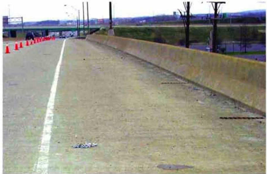
This bridge maintained corrosion resistance at barrier.
