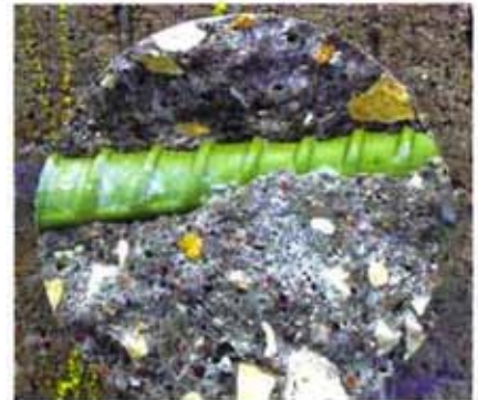
Core sample from bridge showing epoxy-coated rebar in perfect condition.
