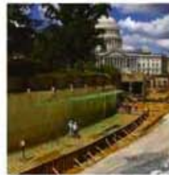
Steel braces stabilize the formwork for a concrete wall in the CVC truck tunnel
