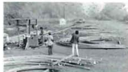
Large rebar radius is apparent in this job-site fabrication set up.
