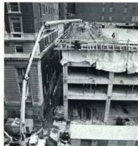
All concrete was pumped for the 8-story garage.
