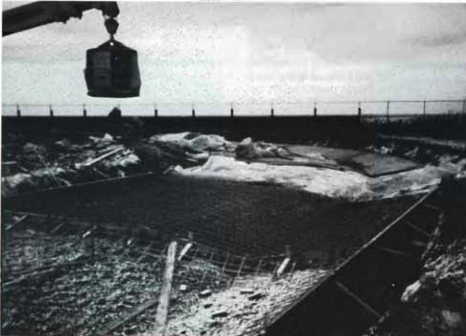
Construction of the large gutter which surrounds the stock pile.
