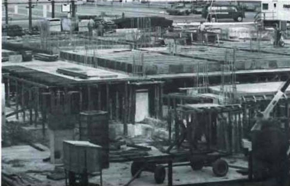
While excavating goes on, epoxy-coated rebar is placed on one level (right) as downward progress starts. ▲
