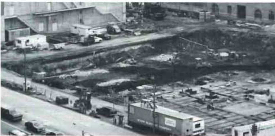
While excavating goes on, epoxy-coated rebar is placed on one level (right) as downward progress starts. ▲
