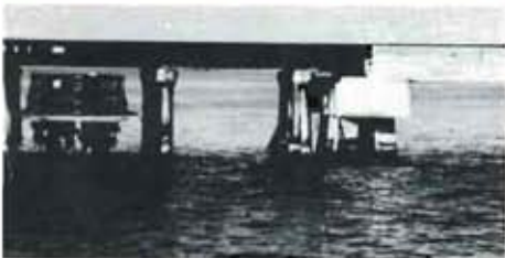
Closeup showing new concrete section adjoining old, original wood span.
