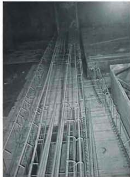
Epoxy-coated rebar cage that will become a girder at P-2 level.
