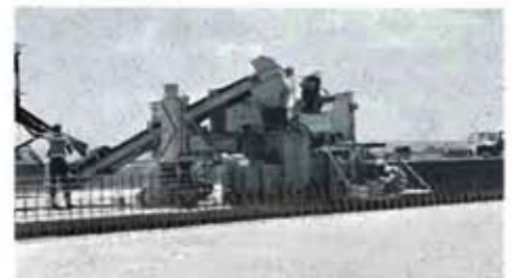
Parapet wall construction moves at a continuous rate with concrete fed to the slipform paver. (Photos courtesy Figg and Muller Engineers, Inc. and Pary, Inc.)
