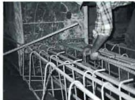
Threaded taper epoxy-coated rebar being installed in epoxy-coated Lenton couplers cast in columns for girder connection at P-2 garage level.
