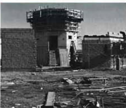
Forming the central core. All rebar is epoxy coated.
