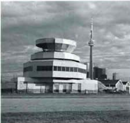
Completed control tower with spiraling CN Tower at right in background.
