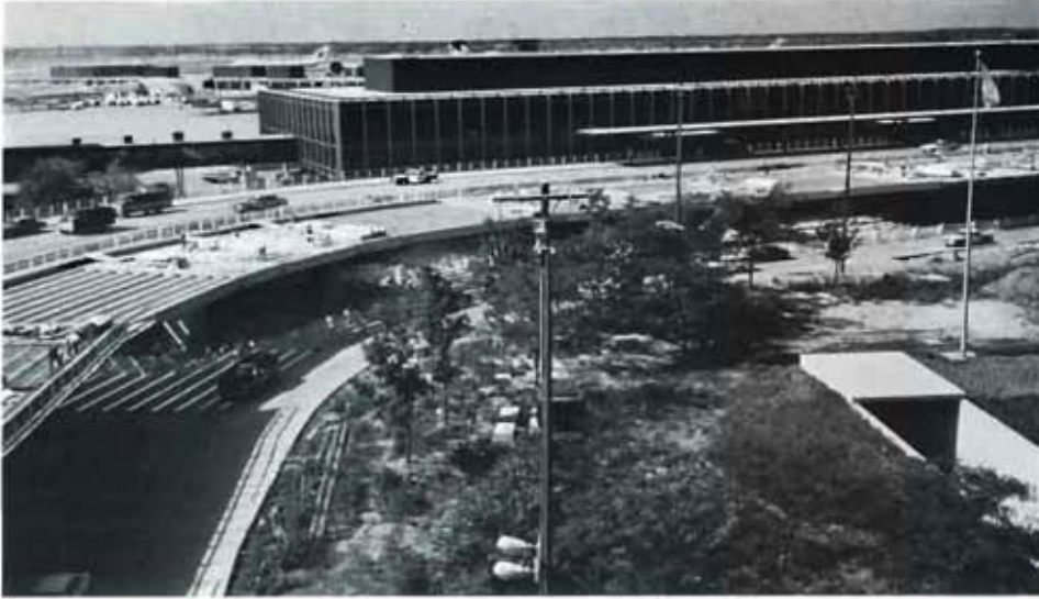
Sweeping around Terminal 2, work progresses on schedule
