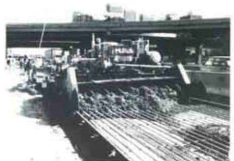
As the Dan Ryan enters the "Loop" area, the roadway returns to grade. Here, the concrete pavement is being placed over the epoxy-coated rebar.
