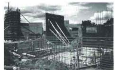
Construction of the huge tank for whales and dolphins.
