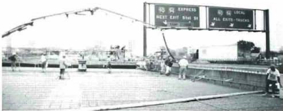
Moving into phase II this year, the contractor paved the northbound bridge deck by pumping concrete from the street below.
