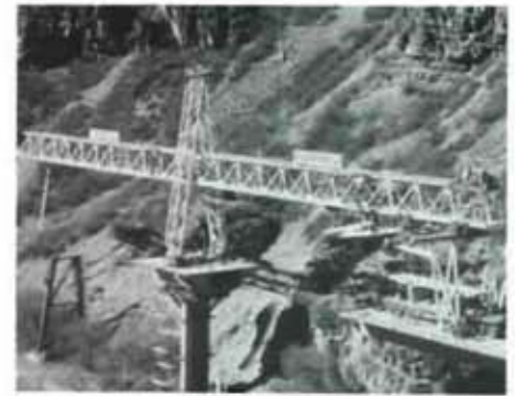
Slow going. Placing segmented section on high pier.
