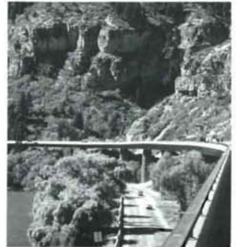
A completed section. Existing I-70 in foreground.
