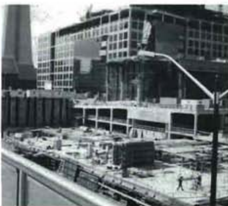
Early construction scene showing garage area where epoxy-coated rebar was specified.
