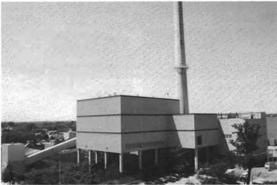
The completed addition to the coal-fired heating plant with large enclosed area housing the filtration equipment. Note the coal piled around the support columns.
