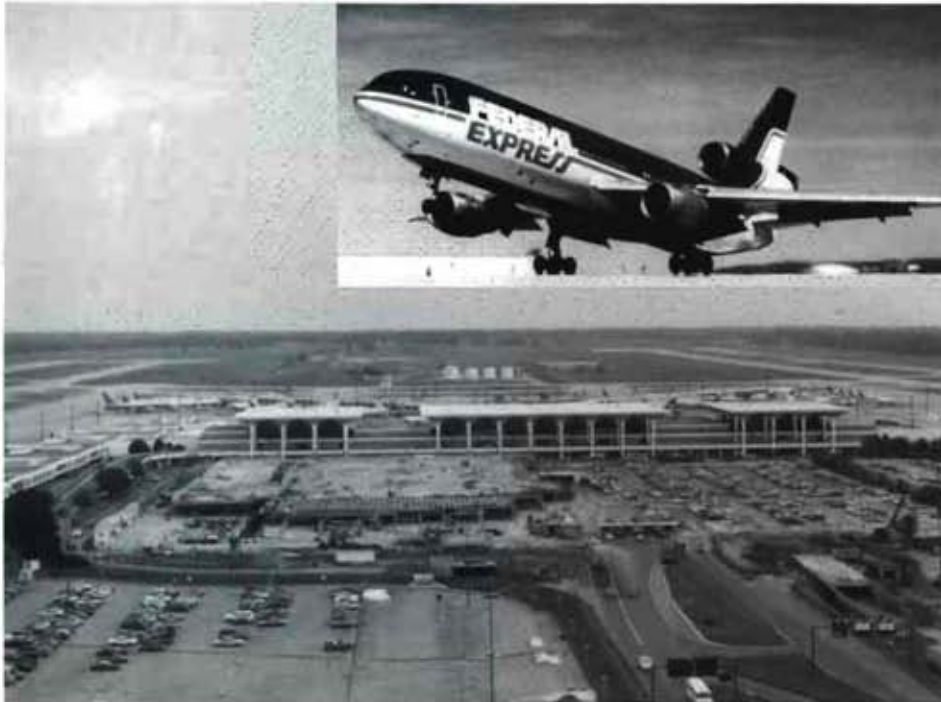
Air view of airport shows construction of parking garage and additional terminal driveway capacity. The airport is a base for eleven passenger airlines and fifteen all-cargo airlines.
